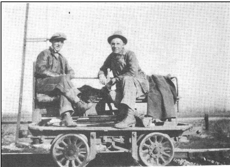
Repairmen's transportation for the Sanpete Railroad tracks.
