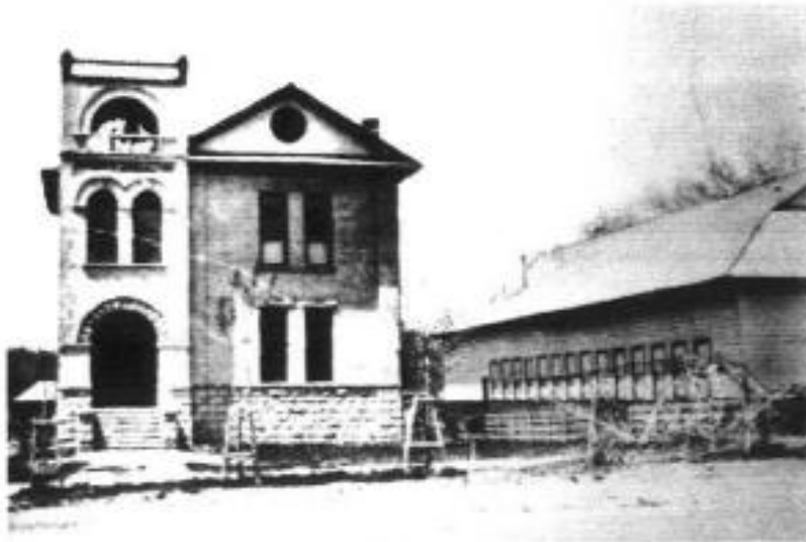
The Garrison City Hall and John S. Peterson Dance Hall on the right.
