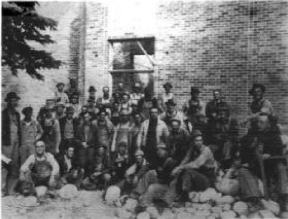
Construction workers on the Manti School.
