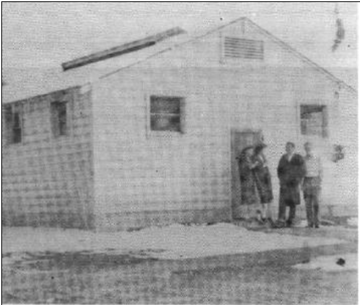
968 used as cafeteria, Union Building, Maintenance Building. Courtesy Snow College
