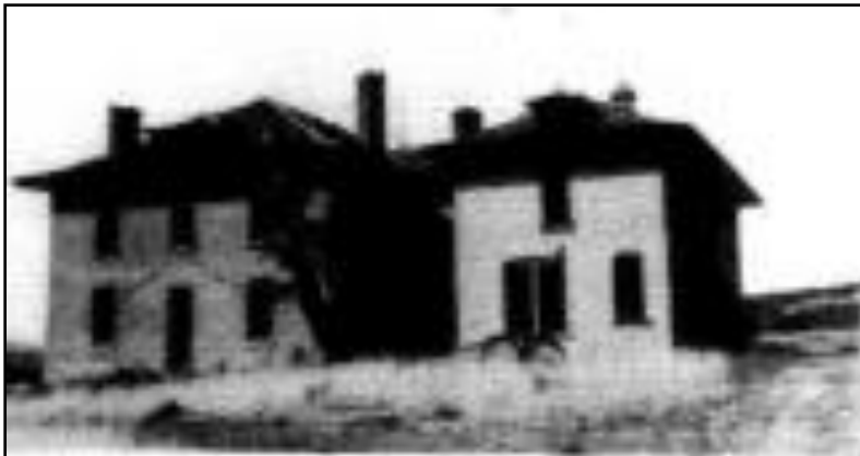
The Infirmary Near Fairview Canyon . See p. 25. Photo-courtesy, Ruth Scow
