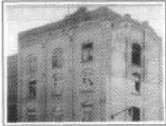
The old Mill in Manti is now under plans for restoration (Picture, Courtesy Lillian Fox)
