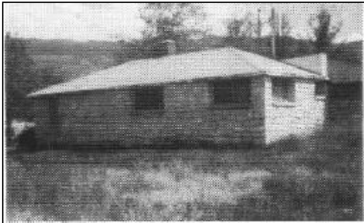
The second floor has been removed from some older homes in Manti but the Pioneers built the foundations to last Picture - Courtesy Lillian Fox
