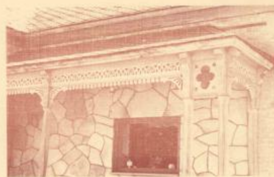
499 South Main — Mantl
